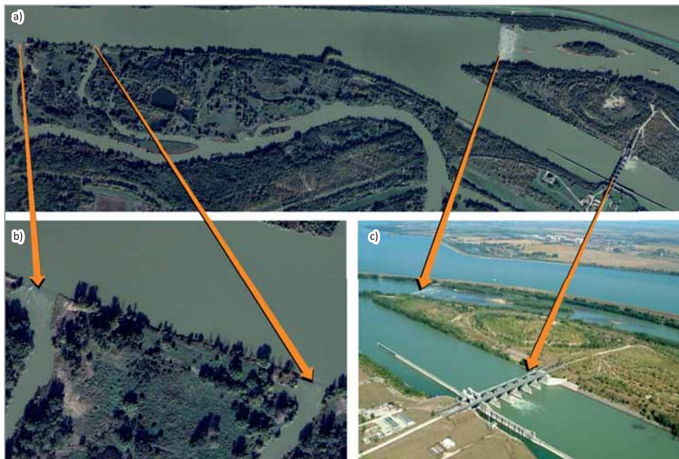
Figure 47: a) Dynamic control of the active floodplain; b) overflow weirs to supply the active floodplain; c) submerged weir, and Dunakiliti Barrage
