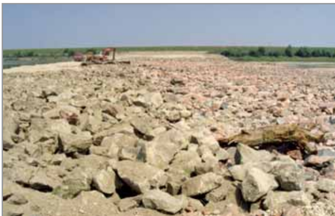
Figure 50: Construction of the submerged weir III
