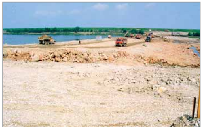
Figure 49: Construction of the submerged weir II
