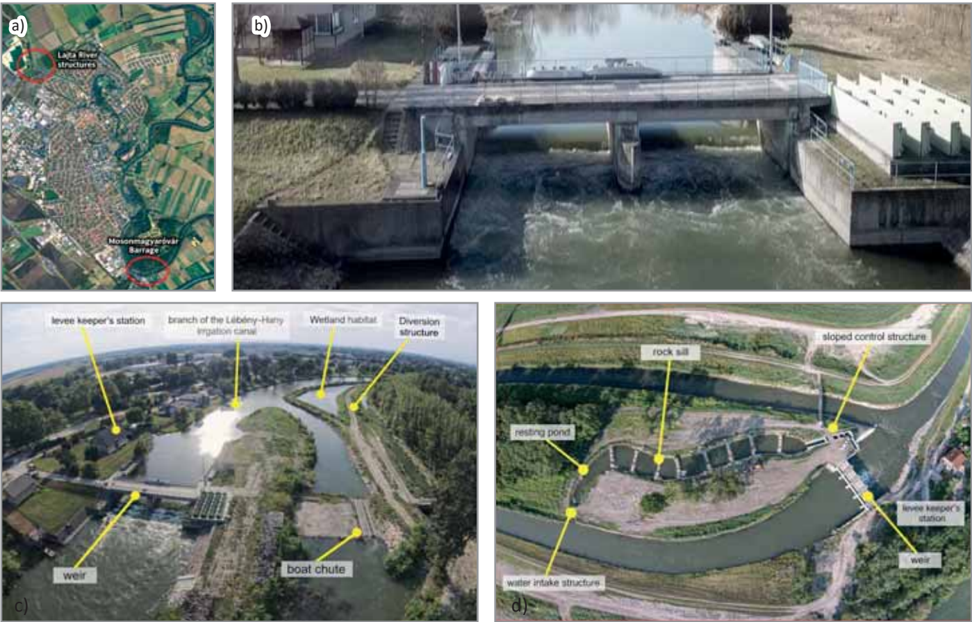
Figure 78: Mosonmagyaróvár Barrage (b, c) and its surroundings on the Mosoni-Danube, and the Lajta control structure and fish passage (d)(Bencze, 2017)
