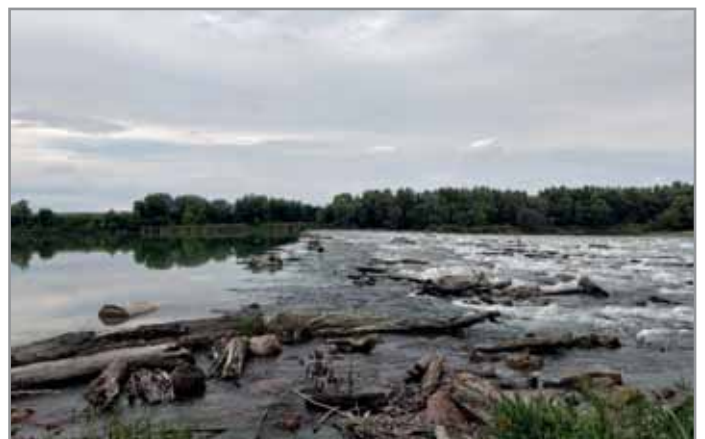
Figure 52: The Dunakiliti Barrage and submerged weir raised upstream water levels, enabling inflow into the active floodplain branch system
