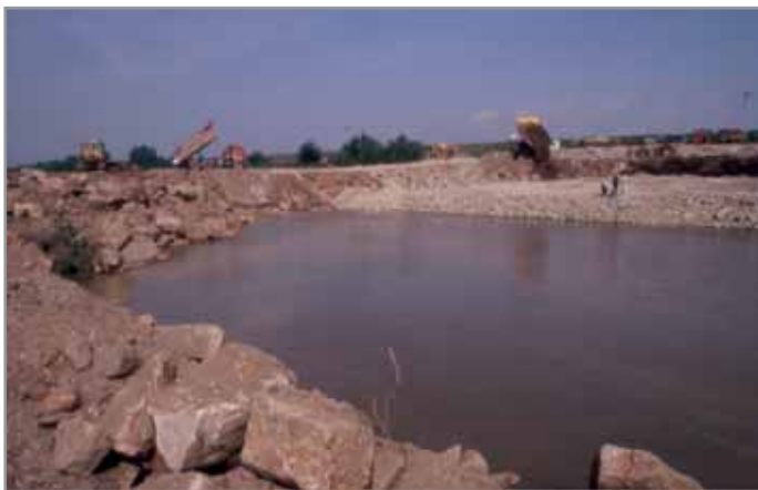
Figure 48: Construction of the submerged weir I
