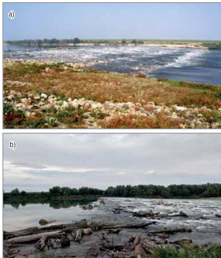
Figure 26: The submerged weir: a) after construction and b) in 2025.
