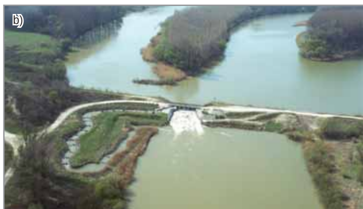
Figure 27: Examples of complex hydraulic structures used to distribute and retain water within the active floodplain: a) “Szent Kristóf” Bridge and water level control structure; b) “Denkpál” branch-end closure and fish passage
