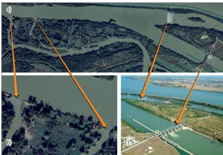
Figure 25: a) Dynamic control of the active floodplain; b) overflow weirs to supply the active floodplain, c) submerged weir, and Dunakiliti Barrage
