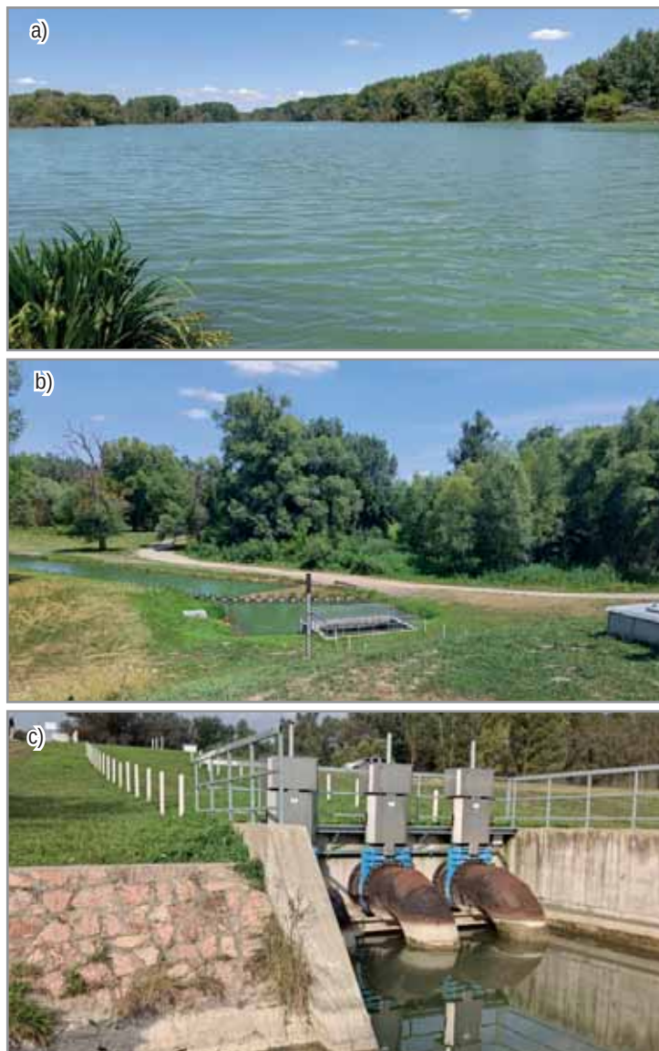
Figure 40: (a) Replenished river branch in Ásványráró; (b,c) Béka-ér Siphon in Ásványráró supplying water from the (b) active floodplain to the (c) historical floodplain
