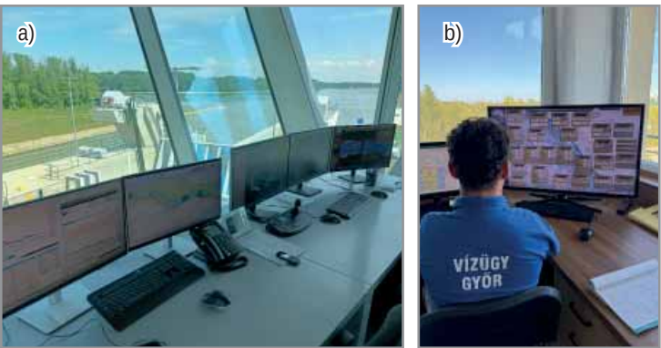
Figure 33: a) Mosoni-Danube outflow structure operation control; b) daily water-level control at Dunakiliti
