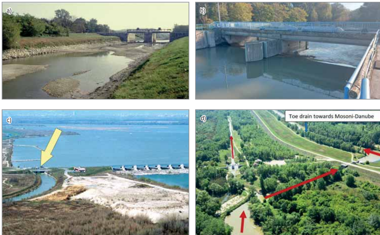
Figure 28: (a) Rajka Sluice Gate in 1991; (b) Mosonmagyaróvár Barrage in 2025; (c) Mosoni-Danube supply channel at the Čunovo reservoir; and (d) flow in the supply channel and toe-drain system near the Rajka Sluice Gate.
